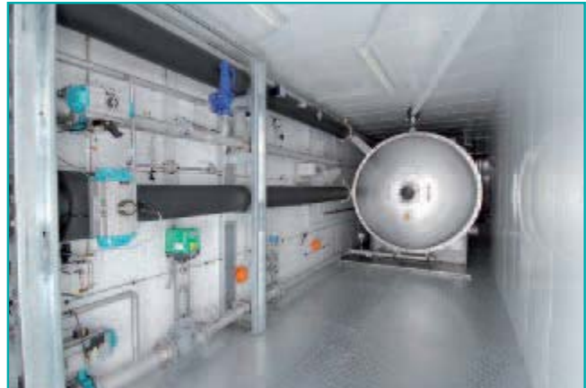
Ozone generator and pipework installed in container
