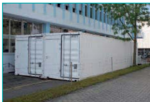
Typical containerised ozone generation systems
