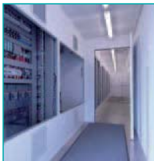
The inside of the container showing the electrical power supply and control equipment
