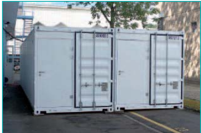
Complete plant seen from the outside
